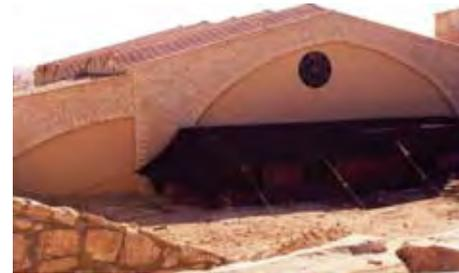
Enclosure over the Church of the Apostles, Madaba, Jordan. The western orientation of the facade and the use of glass resulted in damage to the mosaics from solar radiation, leading to the replacement of the glass with concrete and wooden panels.
