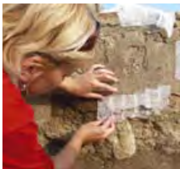
Course participant applying a gauze facing to a render, before its reburial.
