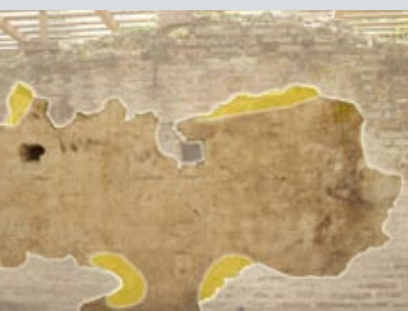
Visual documentation of wall at Sirmium, Serbia. Top: location of cavities in blue; bottom: areas with detachments in yellow
